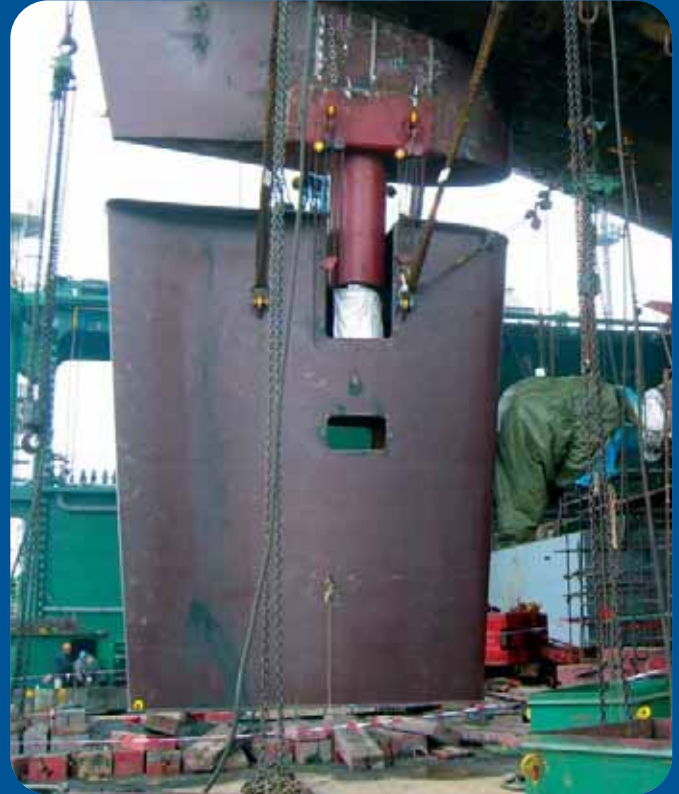
Schilling® KSR Rudder Installation
